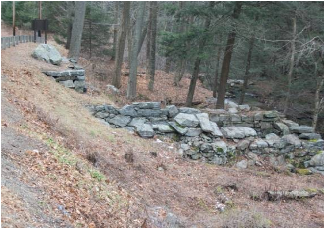
Photograph 1: The Borden's Condensed Milk Factory Site is situated between Burr Mountain Road to the east, and a stream from Burr Mountain Pond to the west. What remains is a terraced fieldstone foundation, a fieldstone wheel pit with a rusted turbine partially buried in it, and brick other artifacts scattered across the surface by the stream.
