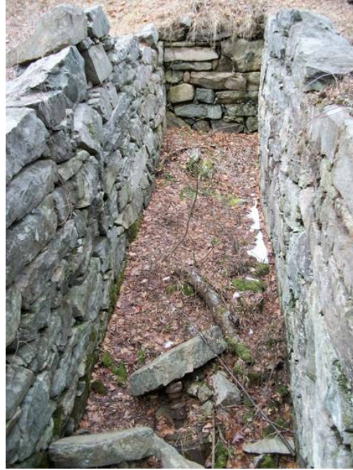
Photograph 2: Inside the wheel pit facing east with the partially buried and rusted turbine visible beneath a slab of cut fieldstone.
