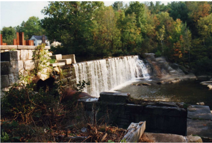
Photo 2: Dam on the Blackberry River that provided power for the Beckley Furnace.
