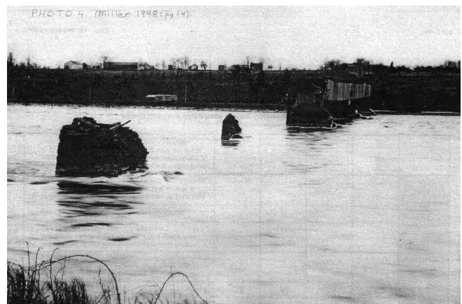
Wreckage of the Enfield-Suffield Bridge in 1900
